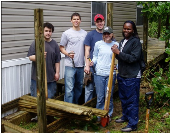
Wheelchair Ramp Build
